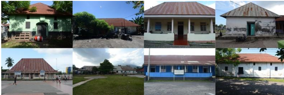
Fig.5.17. Façade of the Buildings inside Fort Oranje Source: Field Survey, 2012
